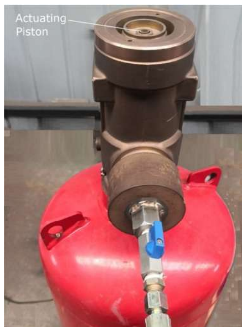
Figure 8.3.4 Actuating Piston
